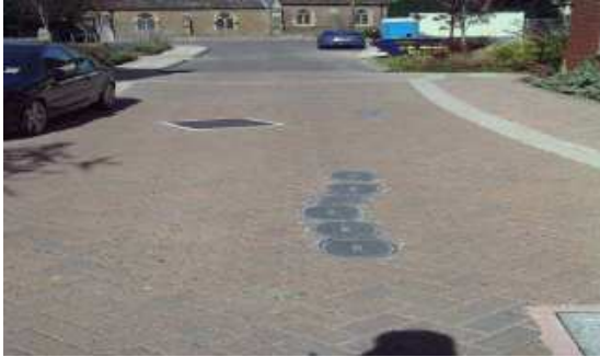
Figure 1 – example of incorrectly installed public utilities on a porous paved road
